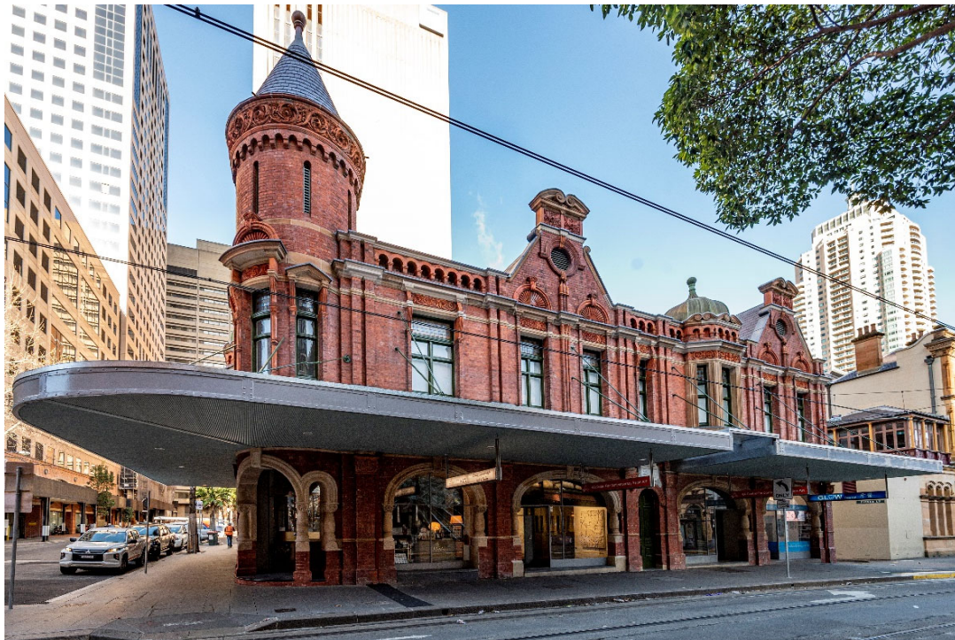
Facing south from Hay Street , Parker Street to the left and Parker Lane to right separating the City owned 744 George St
