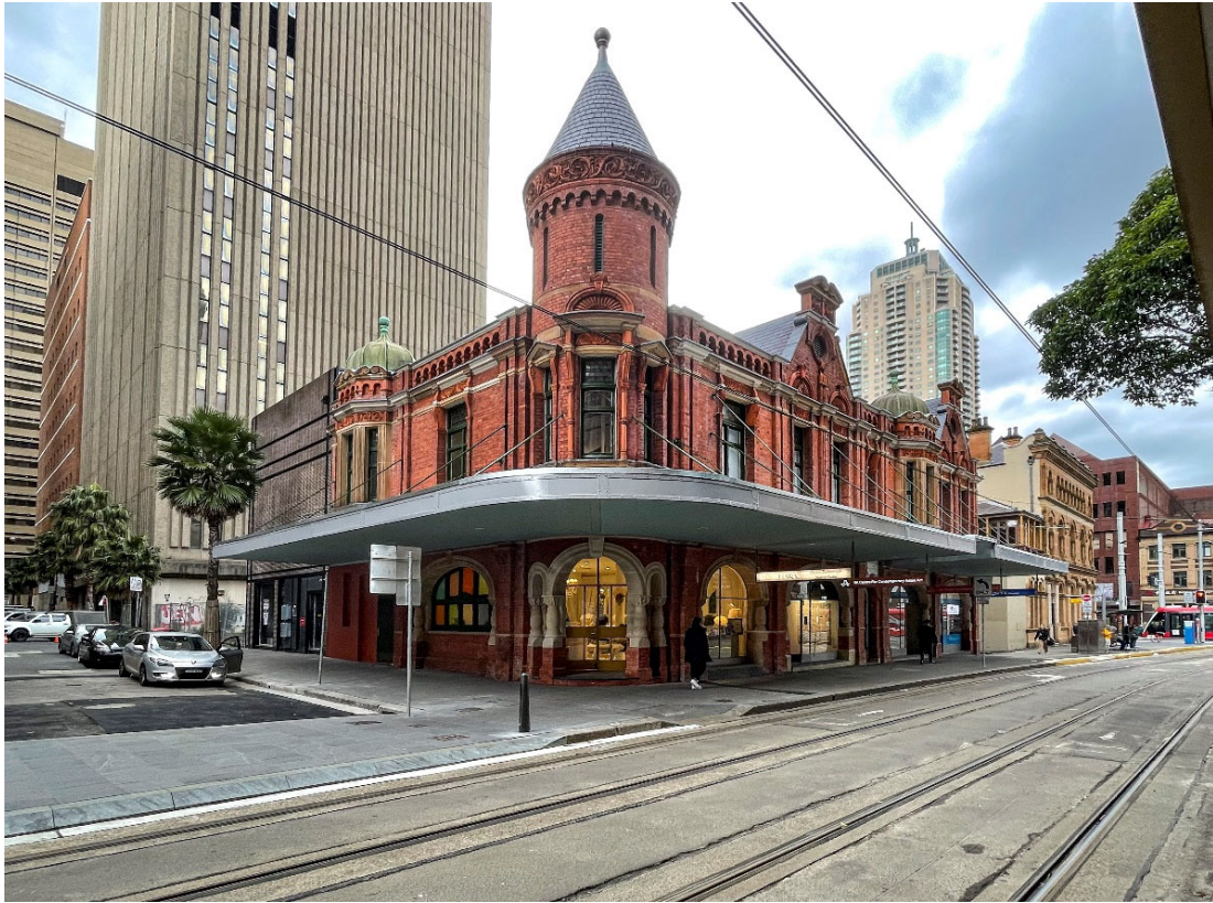
Looking west along Hay Street with Parker Street at left
